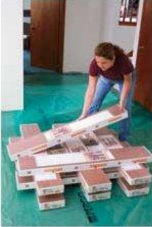
Acclimatize the planks for 48 hours. Two days before you begin work, take the boxes of laminate into the room you're flooring. If applicable set the thermostat at a normal temperature for the time of year. Put the unopened boxes flat on the floor, or stack them three or four high, log-cabin style. After 48 hours, they will have adjusted to the temperature and humidity of the room.
